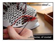
Finally it's time to twist on the wire nuts...
